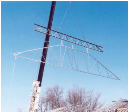
This installer is using a heavy steel truss as a strongback.
