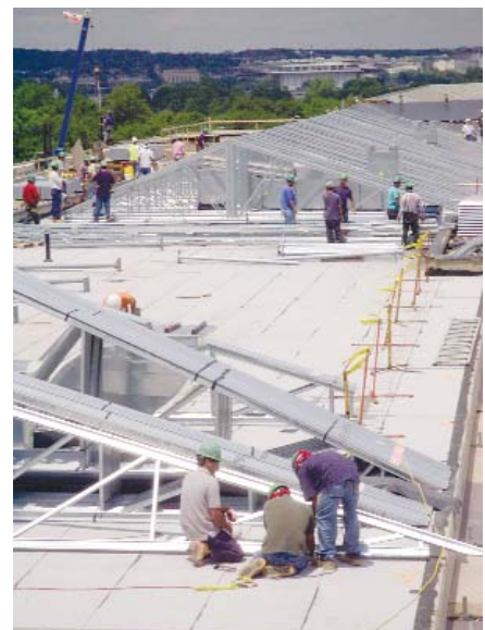
Rebuilding the Pentagon
