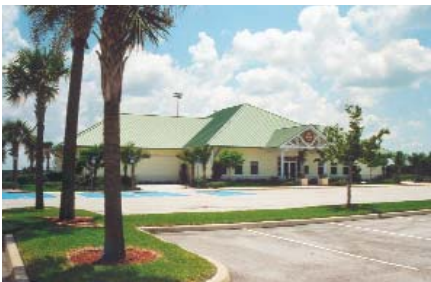
PGA Headquarters, FL
