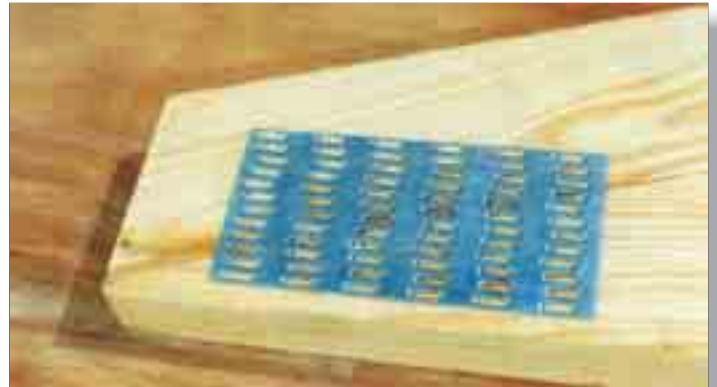
Connector Plate Placement
